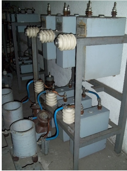
Figure 4.3 Capacitors before Decommissioning
