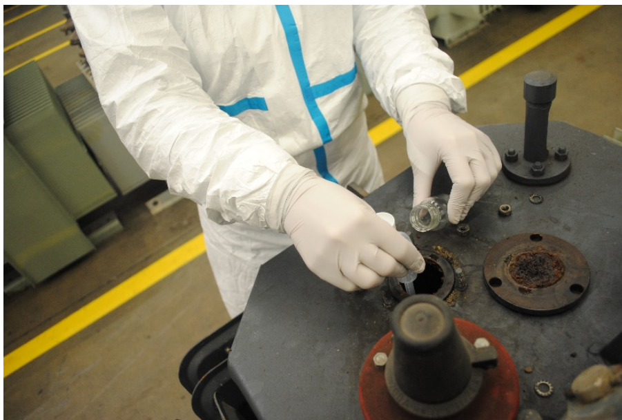
Figure 2.6 Sampling by the Middle of Transformer
